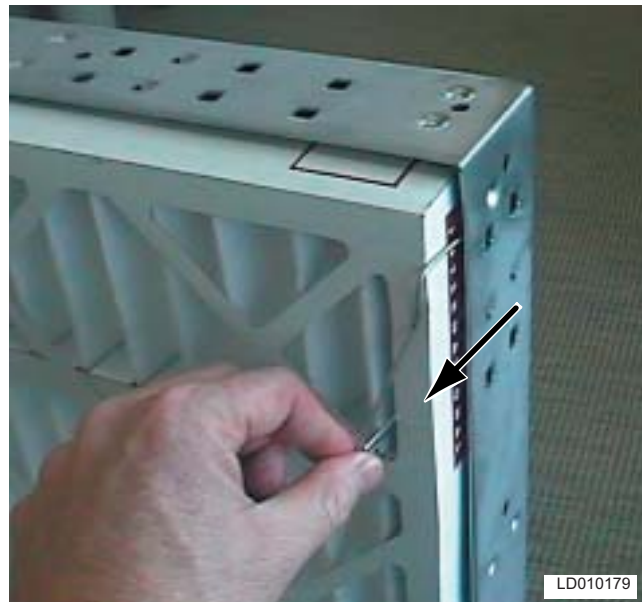
FIG. 36 – PLACE THE END OF THE LATCH OVER THE FILTER FRAME, SECURING THE FILTER TO THE FRAME.
