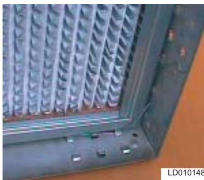
FIG. 37 – FULLY INSTALLED FILTER
