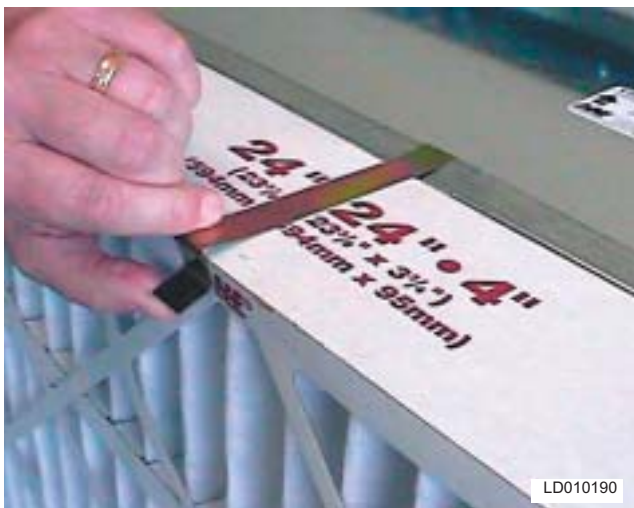
FIG. 48 – SPRING THE END OF THE LATCH SO THAT IT FITS OVER THE EDGE OF THE PREFILTER. (4" W/315-003-004 LATCH SHOWN)
