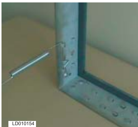
FIG. 41 – CORRECT LATCH/KNOCKOUT CONFIGURATION.
