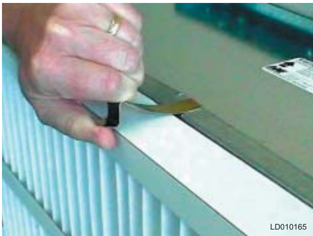
FIG. 47 – POSITION PREFILTER IN FRONT OF THE FINAL FILTER. (2" W/315-003-002 LATCH
