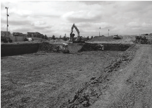
Excavate bed and prepare subgrade per engineer's plans.
