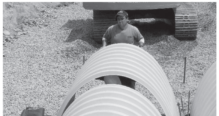
Continue installing chambers by overlapping chamber end corrugations. Chamber joints are labeled "Lower Joint – Overlap Here" and "Build this direction – Upper Joint". Be sure that the chamber placement does not exceed the reach of the construction equipment used to place the stone. Maintain minimum 9" (300 mm) spacing between rows. For the Isolator Row place two continuous layers of ADS Woven fabric between the foundation stone and the isolator row chambers, making sure the fabric lays flat and extends the entire width of the chamber feet.
