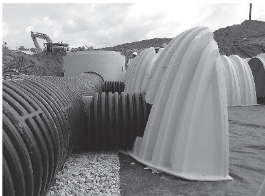
Align the first chamber and end cap of each row with inlet pipes. Contractor may choose to postpone stone placement around end chambers and leave ends of rows open for easy inspection of chambers during the backfill process.
