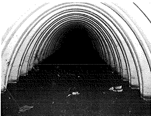
Figure 1 Isolator Row (row 1)
