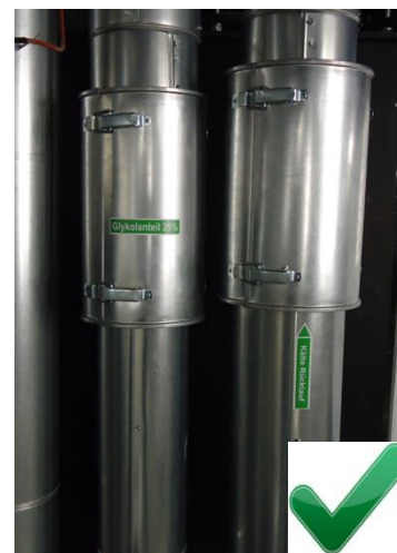
Figure 22 – Insulation with 2 half-shells
