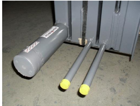
Figure 15 – Heat exchanger drains at time of delivery
