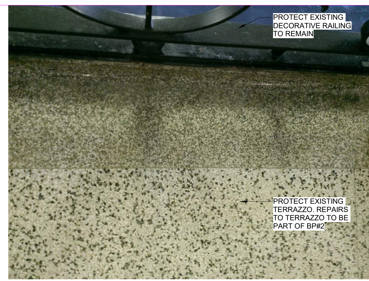
23 TERRAZZO ON GRAND STAIR SD4.22
