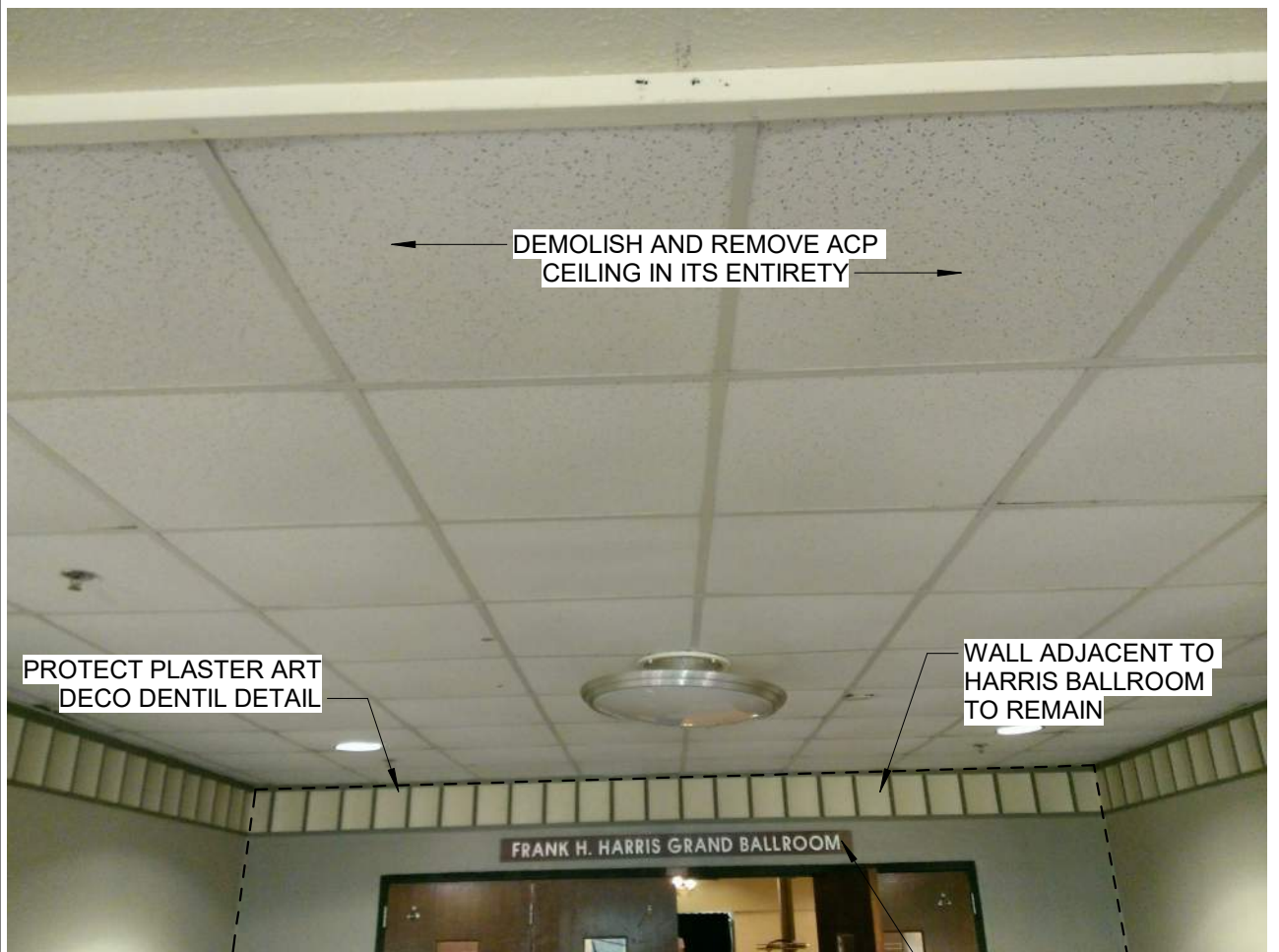
12 CEILING AT ENTRY TO HARRIS BALLROOM SD4.21
