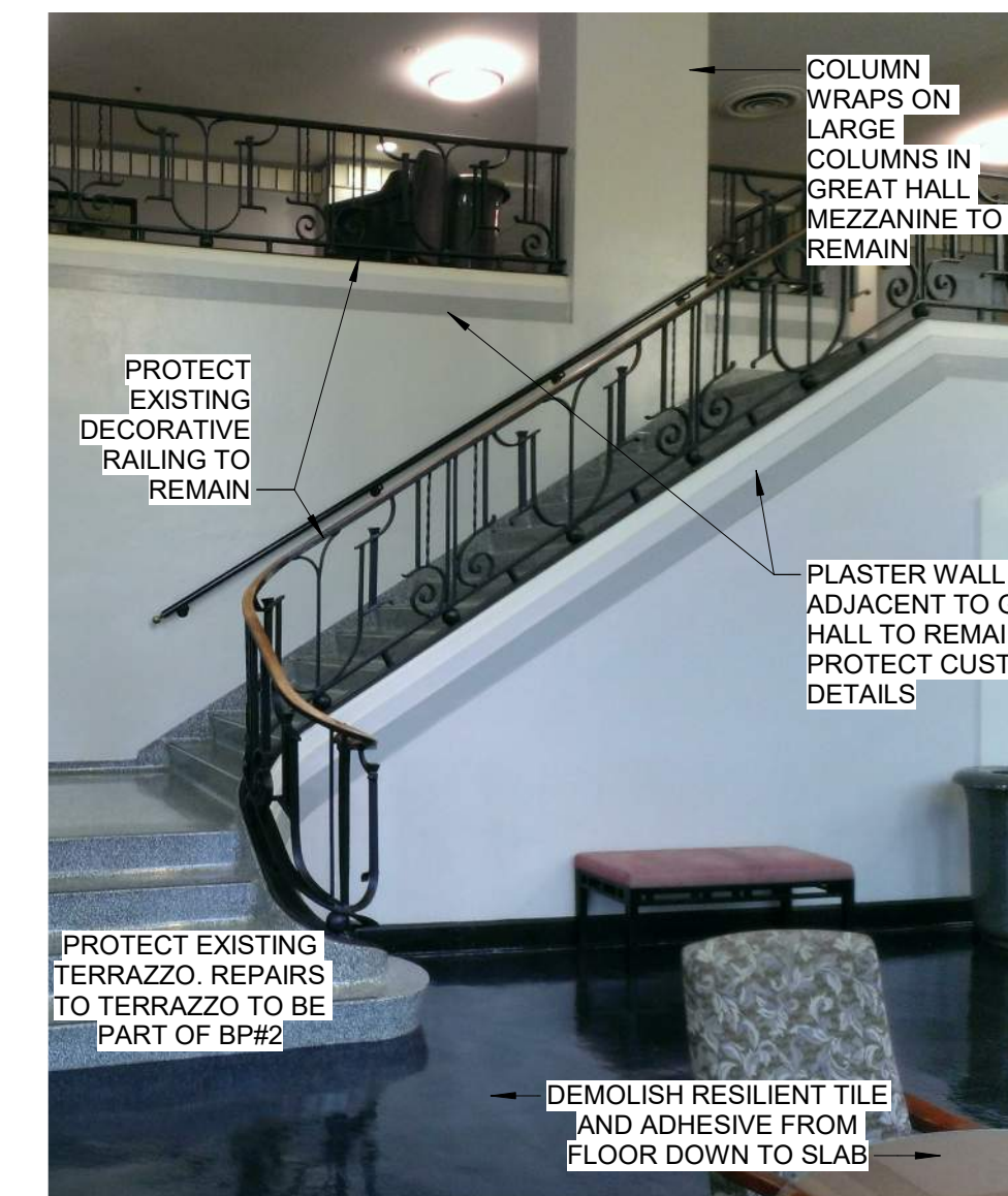
20 RAILING DETAIL AT GRAND STAIR SD4.21
