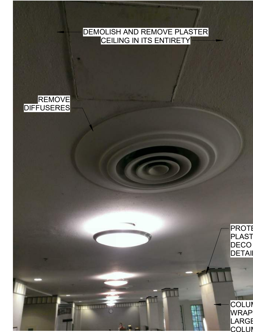
9 CEILING OF GREAT HALL MEZZANINE SD4.21
