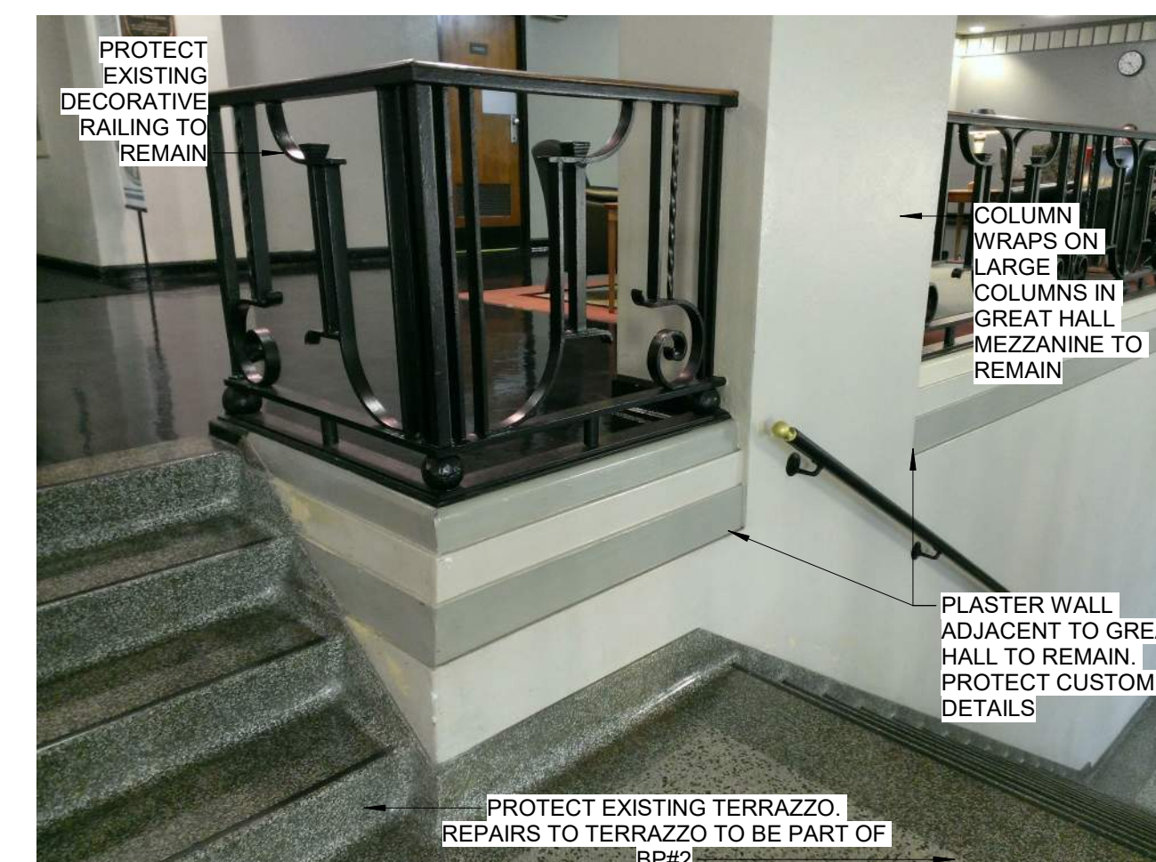
18 RAILING DETAIL AT GRAND STAIR SD4.21
