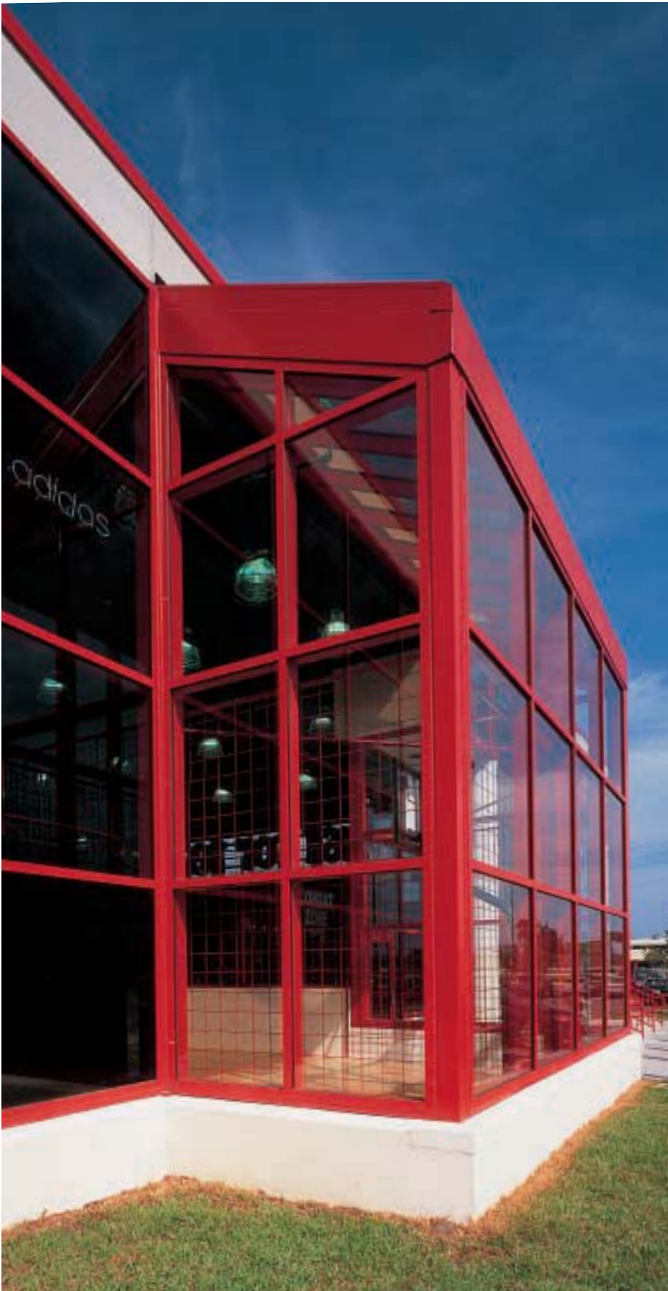
Banner Red Painted Finish Just for Feet, Fort Lauderdale, Fla. Architect: Mark L. Saltz Architects, Inc., Fort Lauderdale, Fla.
