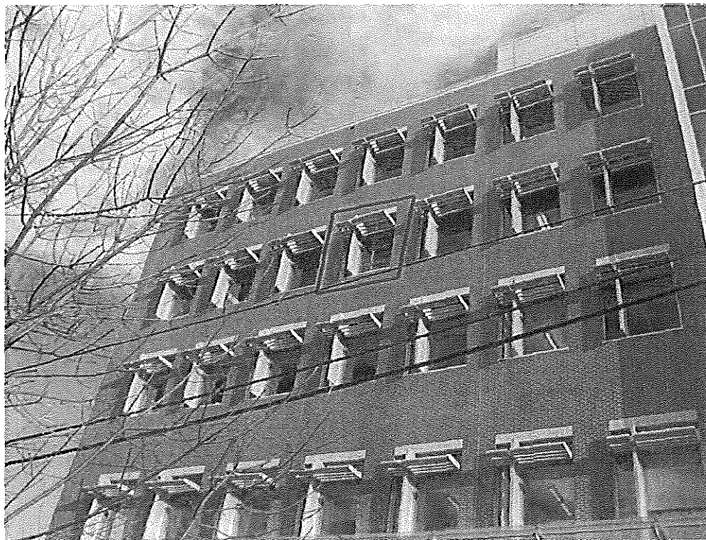
Photo No. 1: Exterior view of Specimen #1
