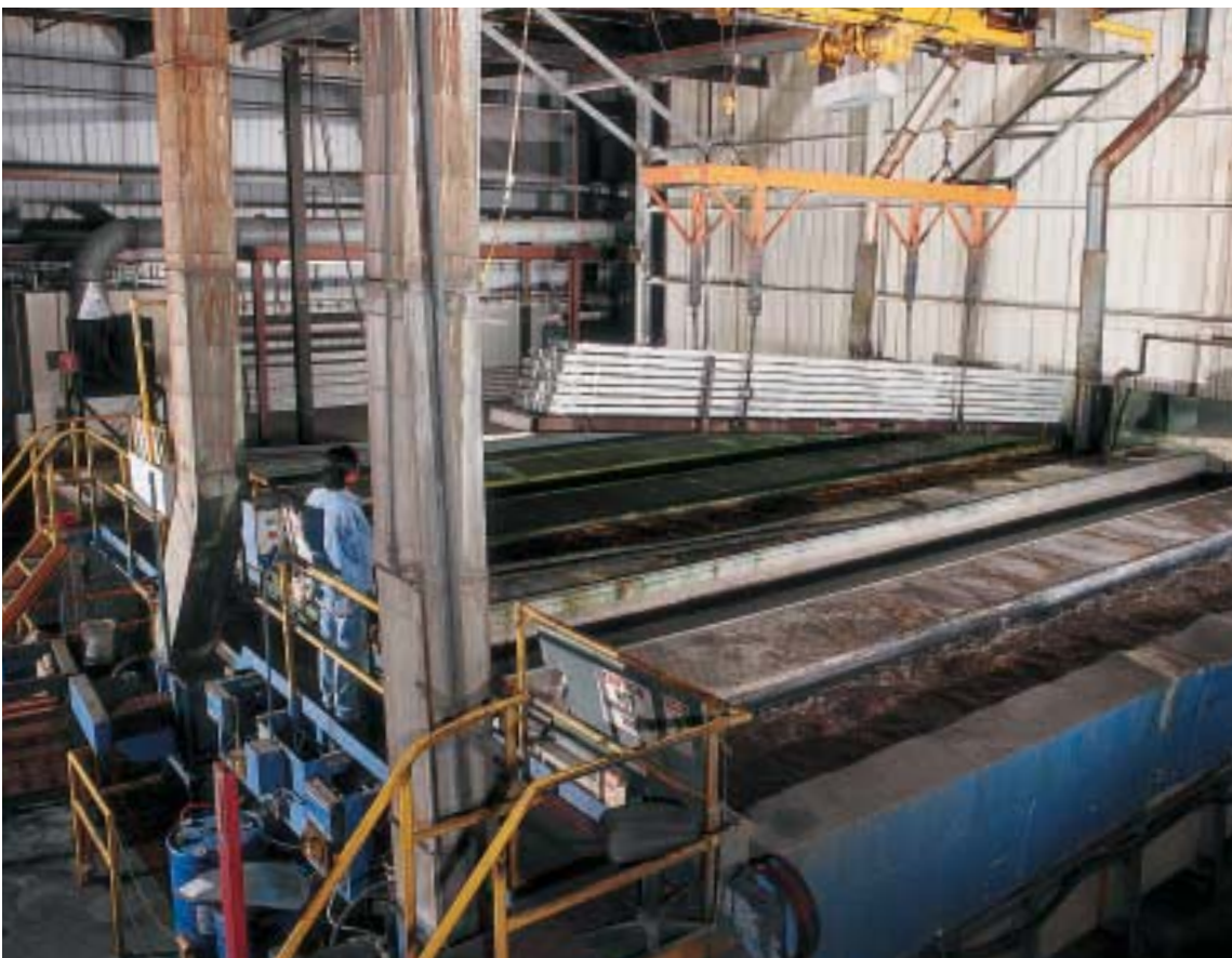
Pre-treatment cleaning processes
