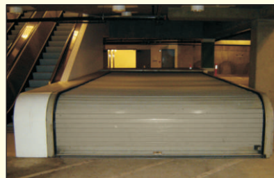
HL250 used for fire and smoke protection in penetrations created by escalators
